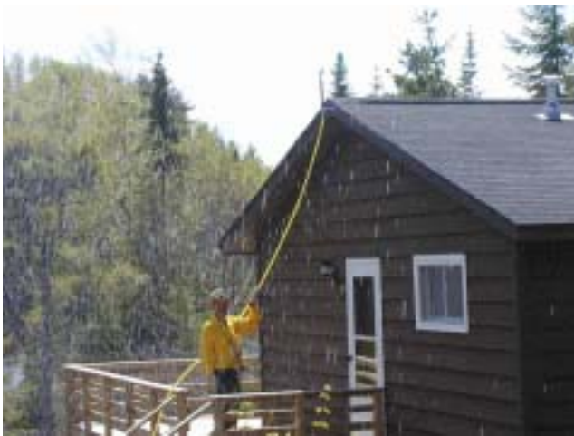
Figure 3.—A member of the Gunflint Trail Volunteer Fire Department developed sprinkler systems to protect homes along the Gunflint Trail, Minnesota.
