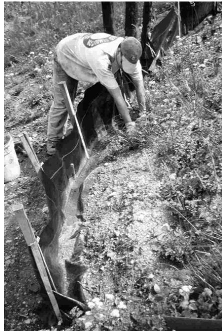
Figure 2. Typical sediment fence where accumulated sediment is being removed (Robichaud 2005).
